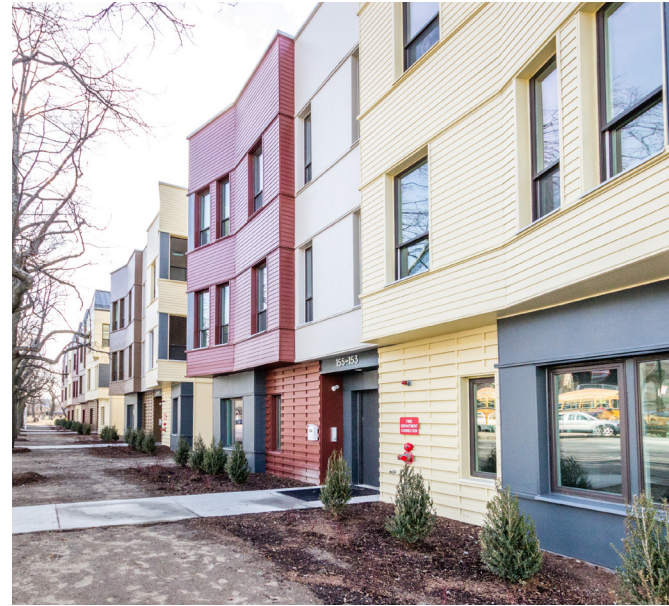
PARCEL U 92 - 171 HYDE PARK AVENUE, JAMAICA PLAIN, BOSTON, MA (Completed)
